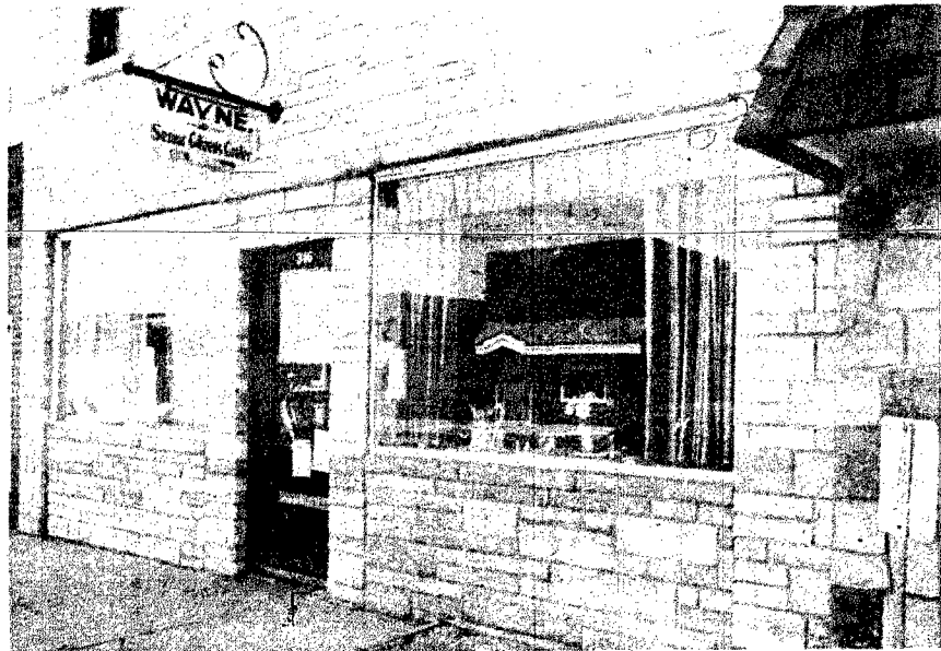
WAYNE'S NEW Industrial site, left photo, serves to attract new industries to the community. The Wayne Senior Citizens Center, above, provides an active program for the city's elderly residents.
